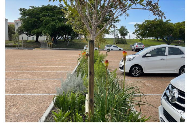
Fig. 6.52. Swales deal with stormwater runoff from hard surfaces
