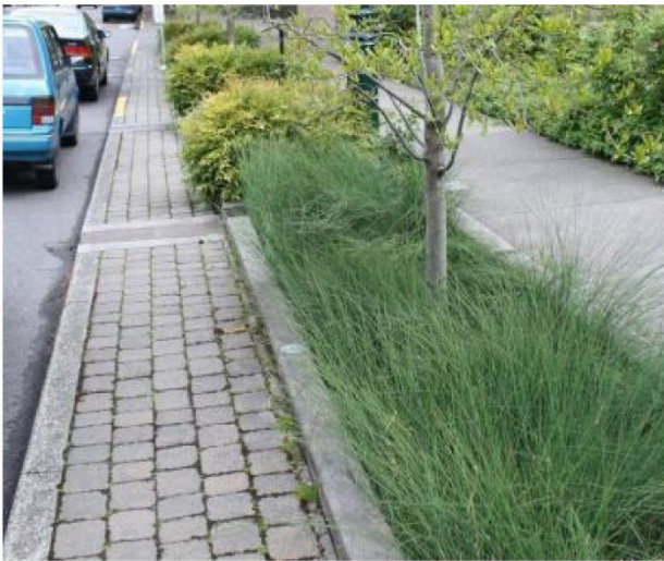
Fig. 6.29. Green street with swale
