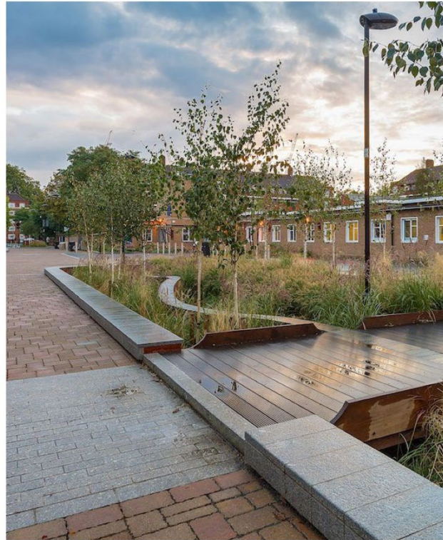
Fig. 6.31. Pedestrian oriented street and shared surface space with Sustainable Urban Drainage System / swale
